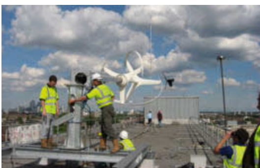
Installation of the new wind turbines
