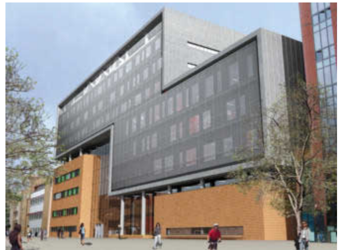
London South Bank University's new Keyworth II building.
