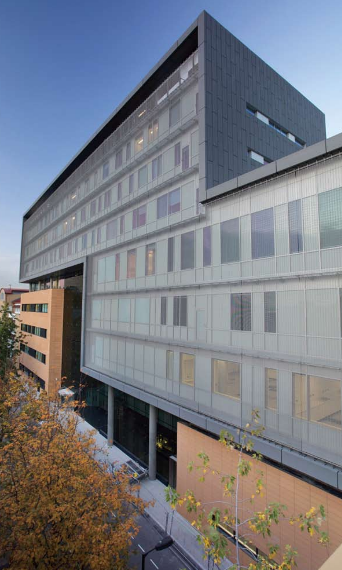
K2 building (opposite), c.2009 Borough Polytechnic Institute, c.1892
